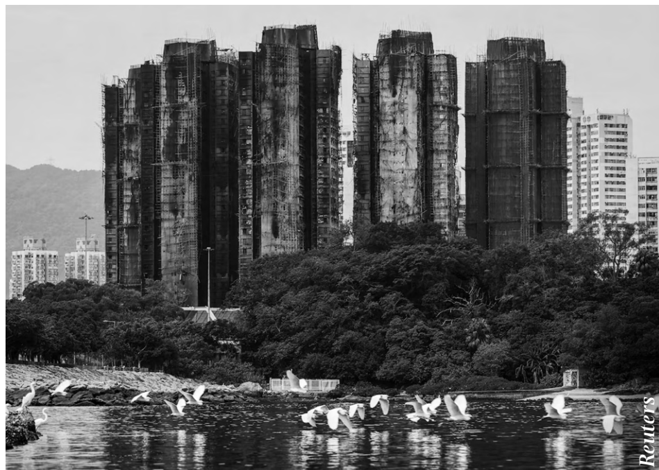
Fire decimates the Wang Fuk Court complex.
