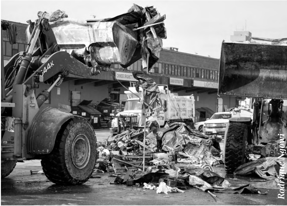
Public works employees bulldoze Mass and Cass residences.
